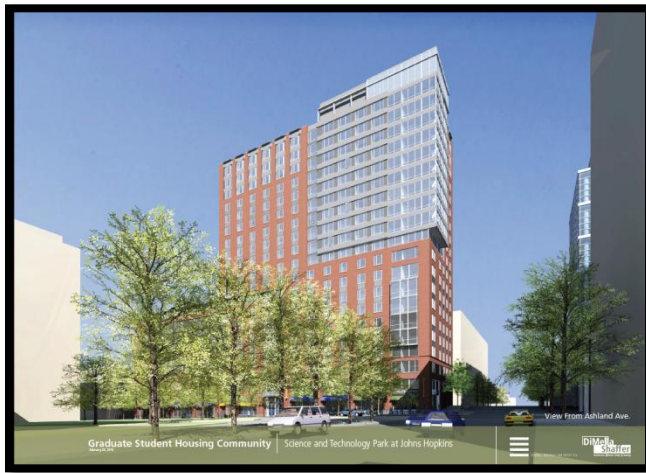
Figure 1 - Showing glass and brick facade along with curtain wall
